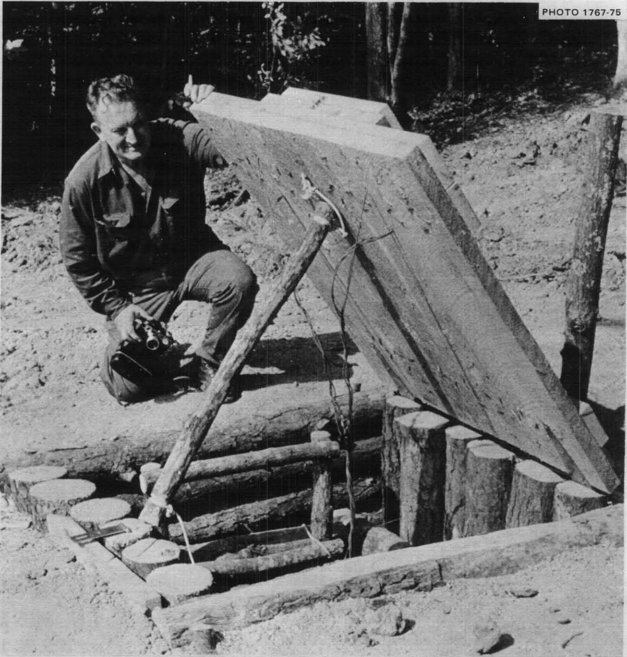
Fig. 7.4. One of the two completed vertical entries, with its expedient blast door made of 2-in.-thick rough lumber. Its hinges were made of strips of worn auto tires, spiked to each of the vertical entryway posts on the hinged side. A door of this type successfully withstood a blast overpressure of 17 psi.* The other blast door was made of 3-in. planks and may have been able to withstand higher blast over pressures than would collapse the earth walls of this covered-trench shelter.
